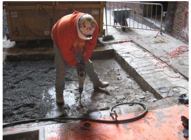
Subgrade for Post Alley Cobblestones
