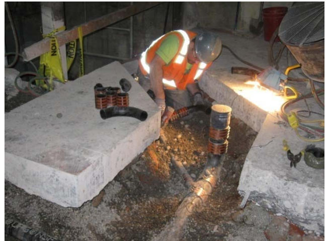
Soames Dunn Bathroom Plumbing Rough-In
