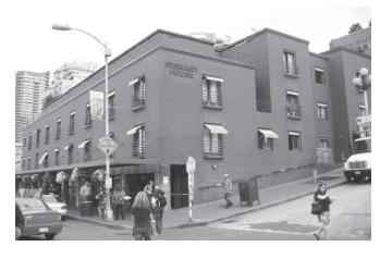
Stewart House renovation plans include removal and replacement of the brick siding; repair of roof; replacement of courtyard pavers and waterproofing; new paint, windows and flooring in apartments; new lights and paint in hallways. For a detailed work plan about this project, visit www.pikeplacemarket.org/renovation/tenant\_information
