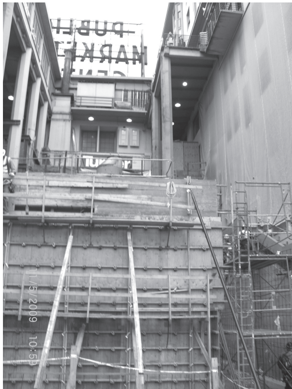
The concrete forms on the Hillclimb.
