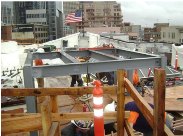
Top of the Elevator Shaft-Corner Market
