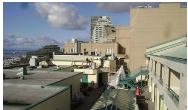
Stucco Work on North Shaft Sanitary Roof
