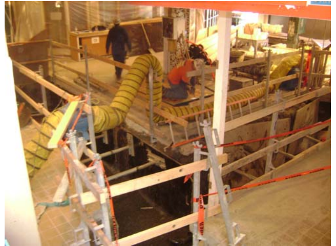
Main Plumbing Trench Sanitary Market
