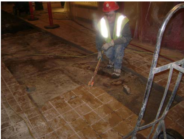
Main Plumbing Trench Sanitary Market
