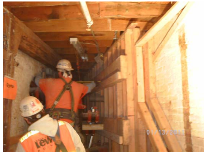
South Point - Structural Upgrades to Triangle Market – Gyro
