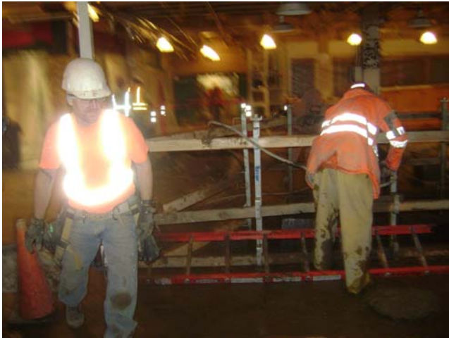
Main Plumbing Trench Sanitary Market
