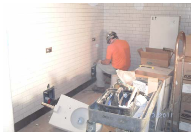
Toilet Install Women's Public Bathroom 602
