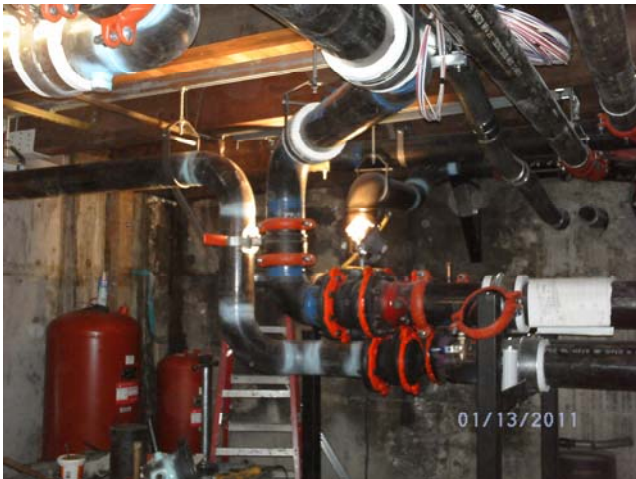
Sanitary Market Basement
