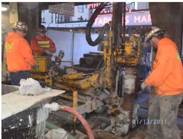
MicroPile Drilling in the Corner Market for Cabbage Brace Frame
