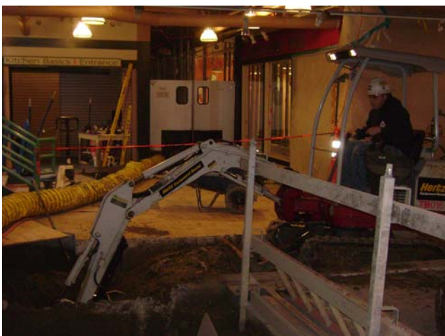
Excavation of the Sanitary Market Trench
