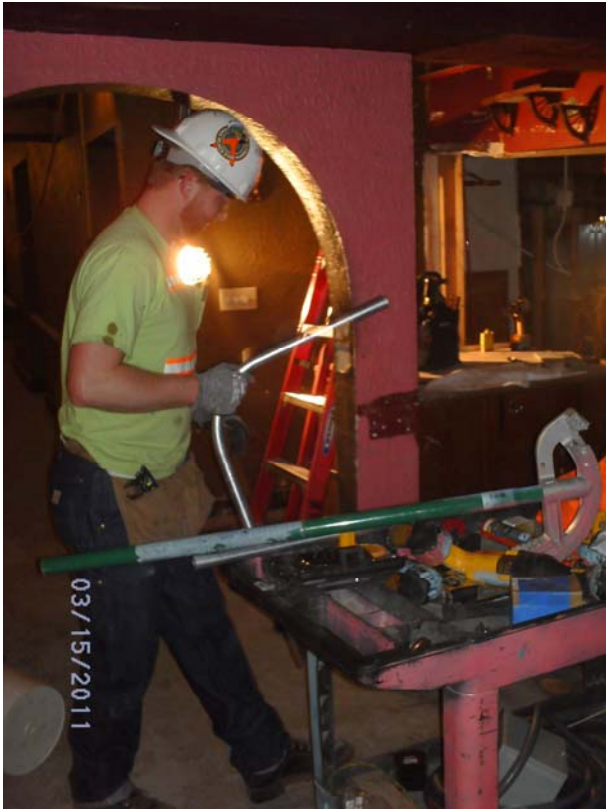
Can Can Electrical Rough-In
