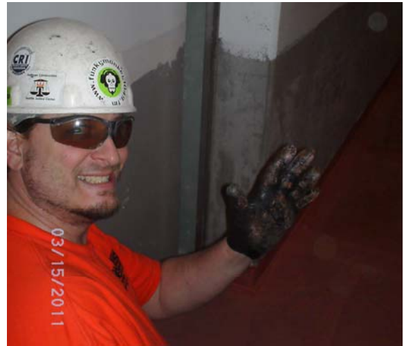
Prepping for Tile Work in 702 Bathroom
