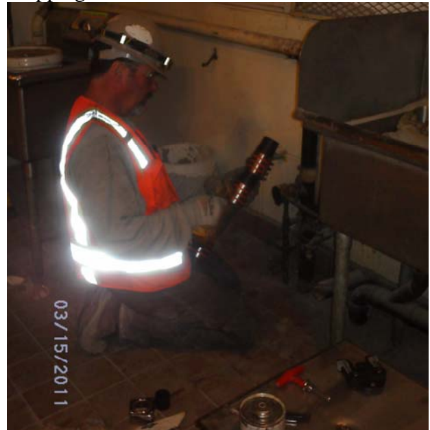
Gary's Snack Shack Plumbing Rough-In
