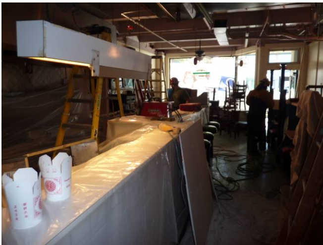
Bayou Grease Shaft work
