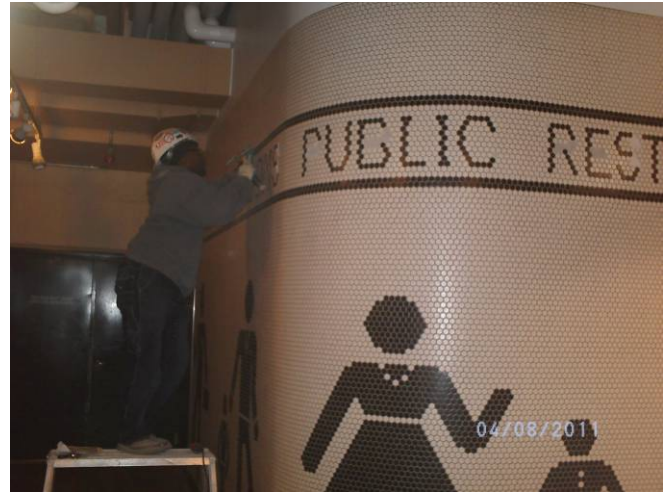
Tile repairs outside 602 bathrooms
