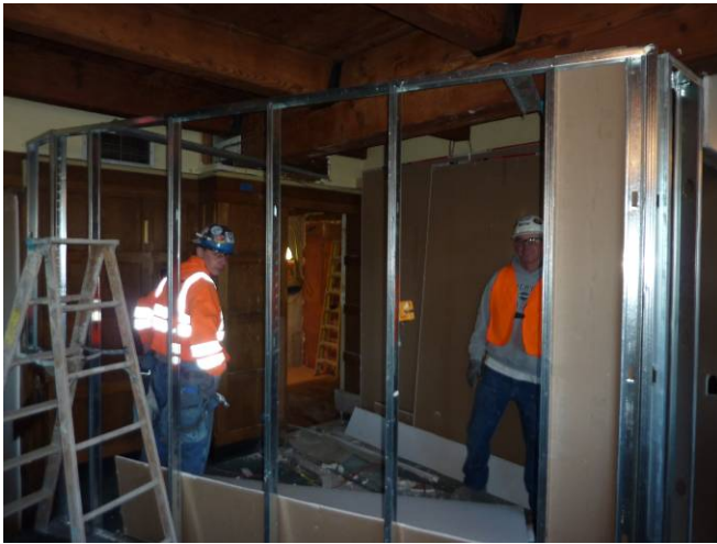
Temp Wall reconfigurations
