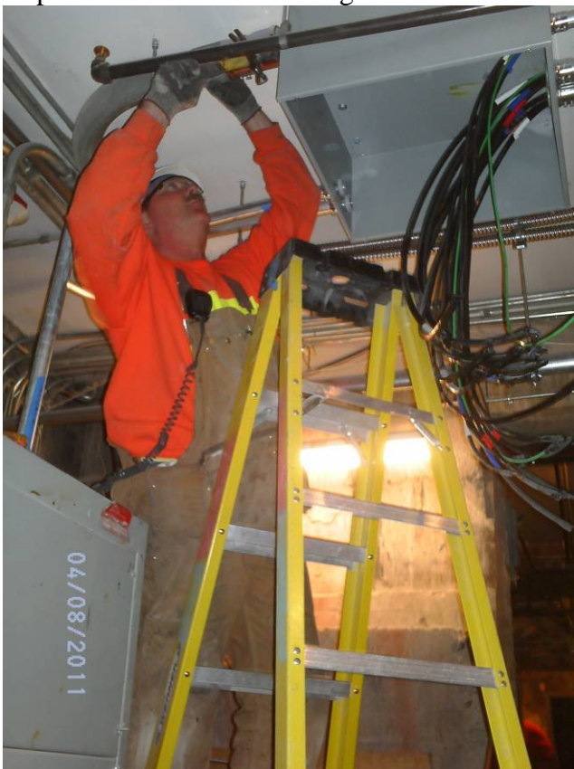
Triangle Basement Electrical Rough-In
