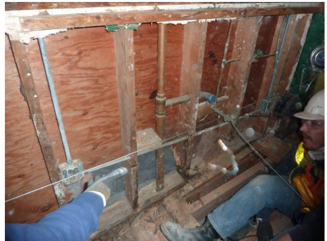
Plumbing Rough In Sanitary Apartments
