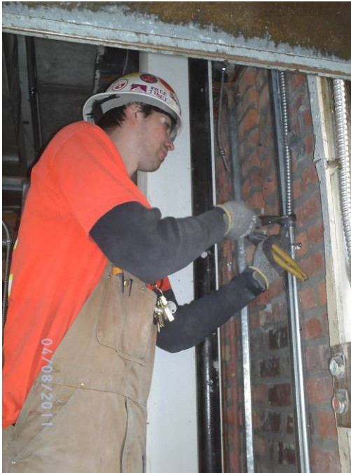
Copacabana – Electrical Rough-In
