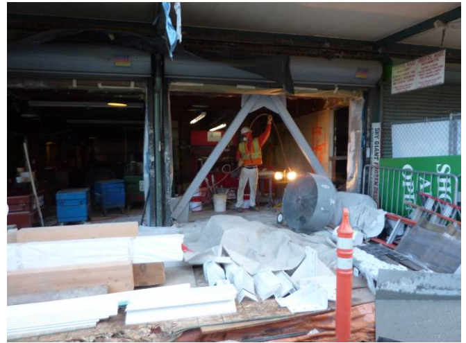
Corner Market – Cabbage Fireproofing
