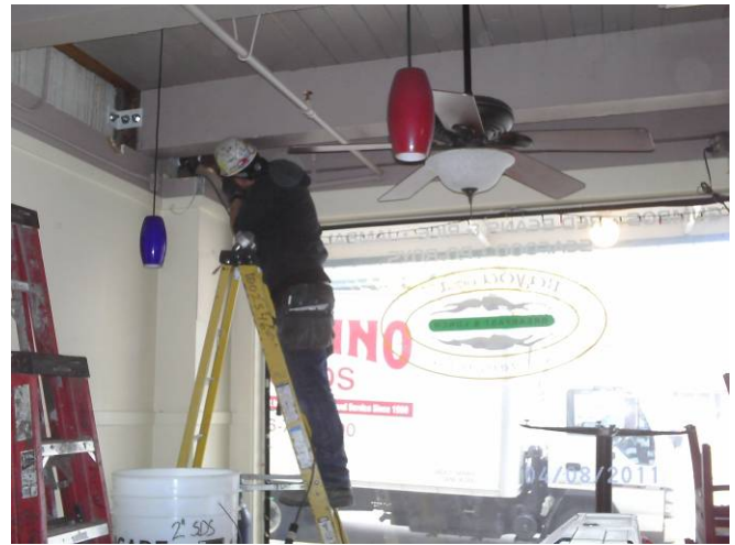
Bayou – drag strut installation
