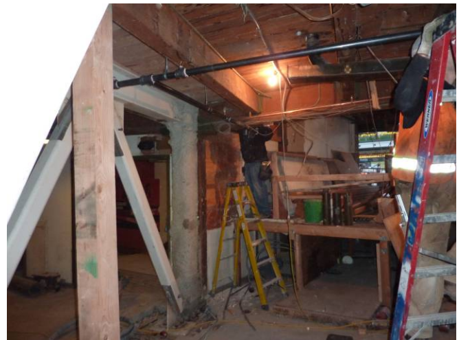
Corner Produce Cooler Prep work
