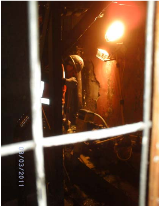
Plumbing Trench near coolers in Sanitary Market
