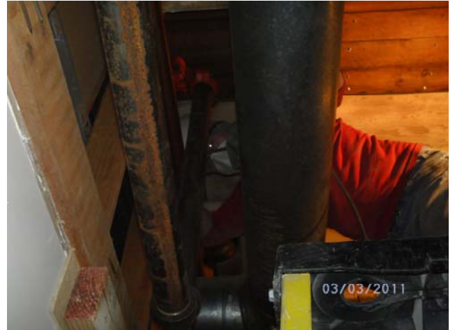
Pipe Fitting on Level 7 of the Sanitary Market
