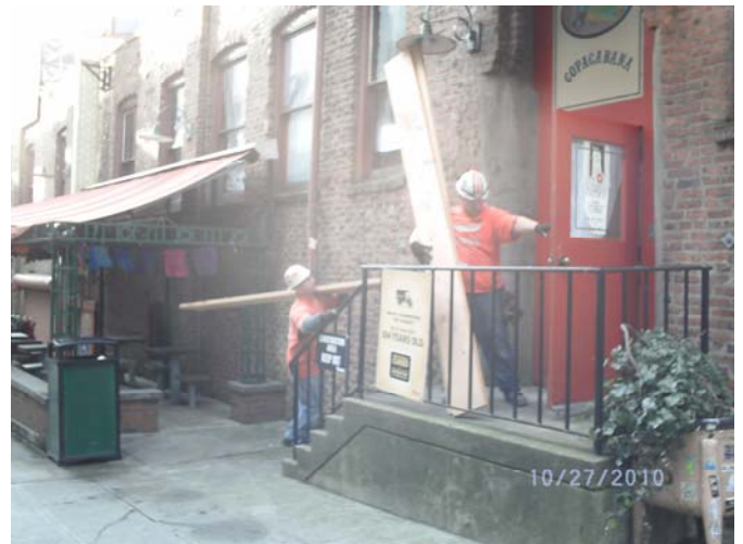
Triangle Market flooring build back
