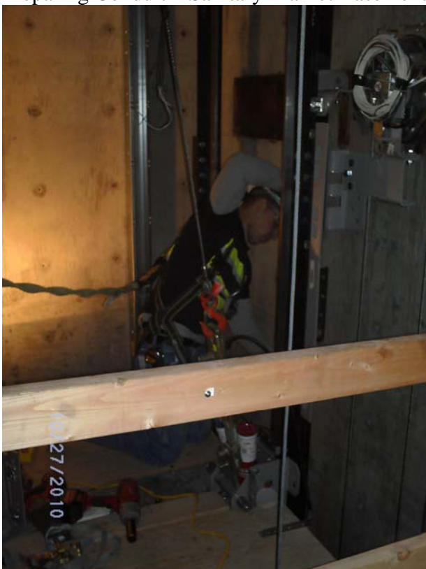
Fine tuning rails elevator shaft – Corner Market
