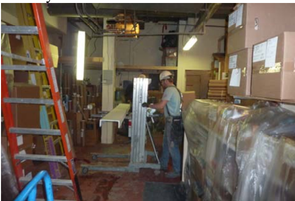
Metsker Maps Drag Strut Installation
