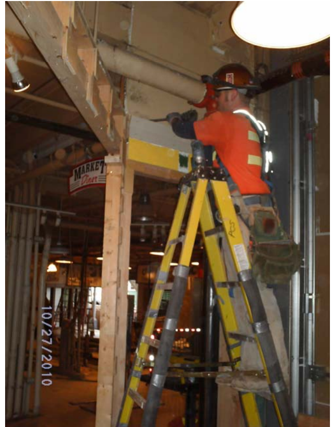
Demolition of wall outside Market Diner
