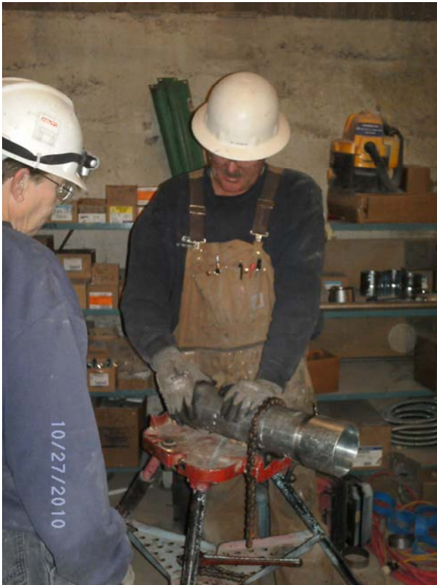
Preparing Conduit – Sanitary Market Basement
