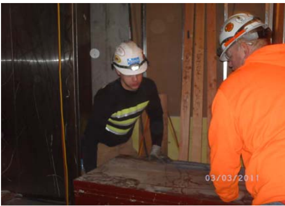
L7 Elevator Lobby
