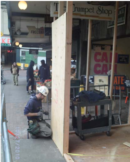
Building Temp Wall outside Left Bank Books
