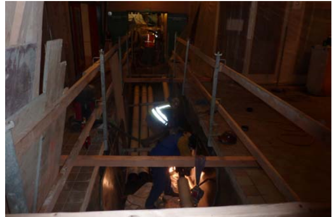
Running Condenser pipes in the Sanitary Market Trench
