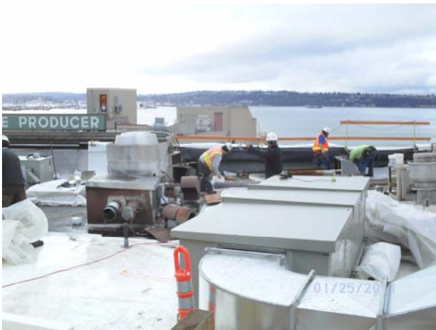
Work on the Corner Market Roof
