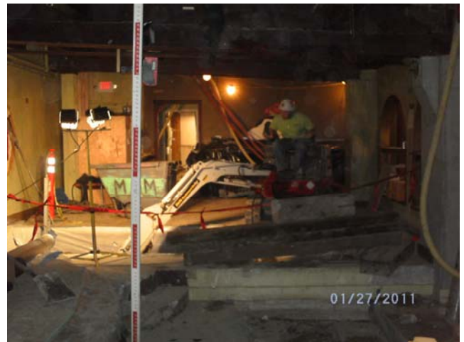
Trenching in tight quarters in Can Can
