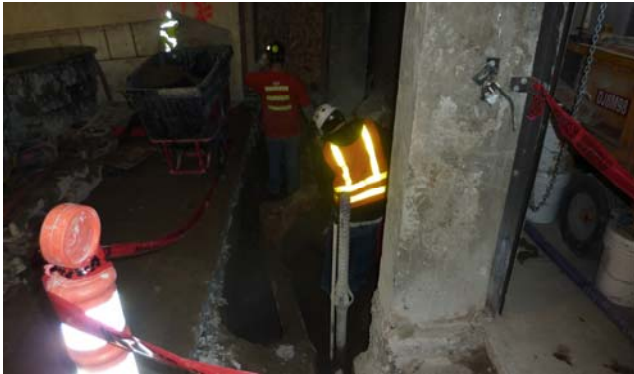
Trenching in the Corner Market
