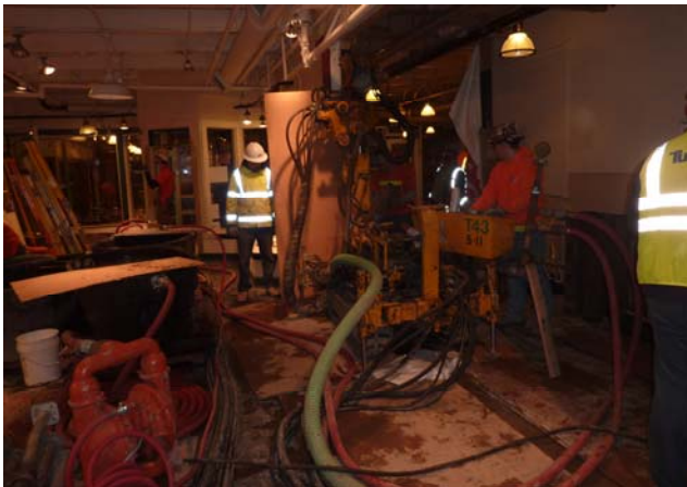
Drilling in Sanitary Market
