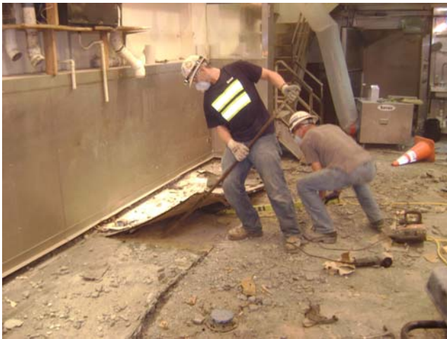
Demolition continues on Pure Food Fish Floor
