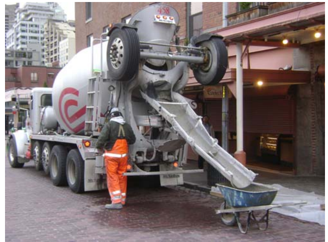
Concrete delivery for Corner Market
